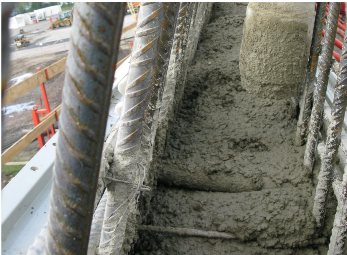
Figure 10 – Concreting the first strap - detail
