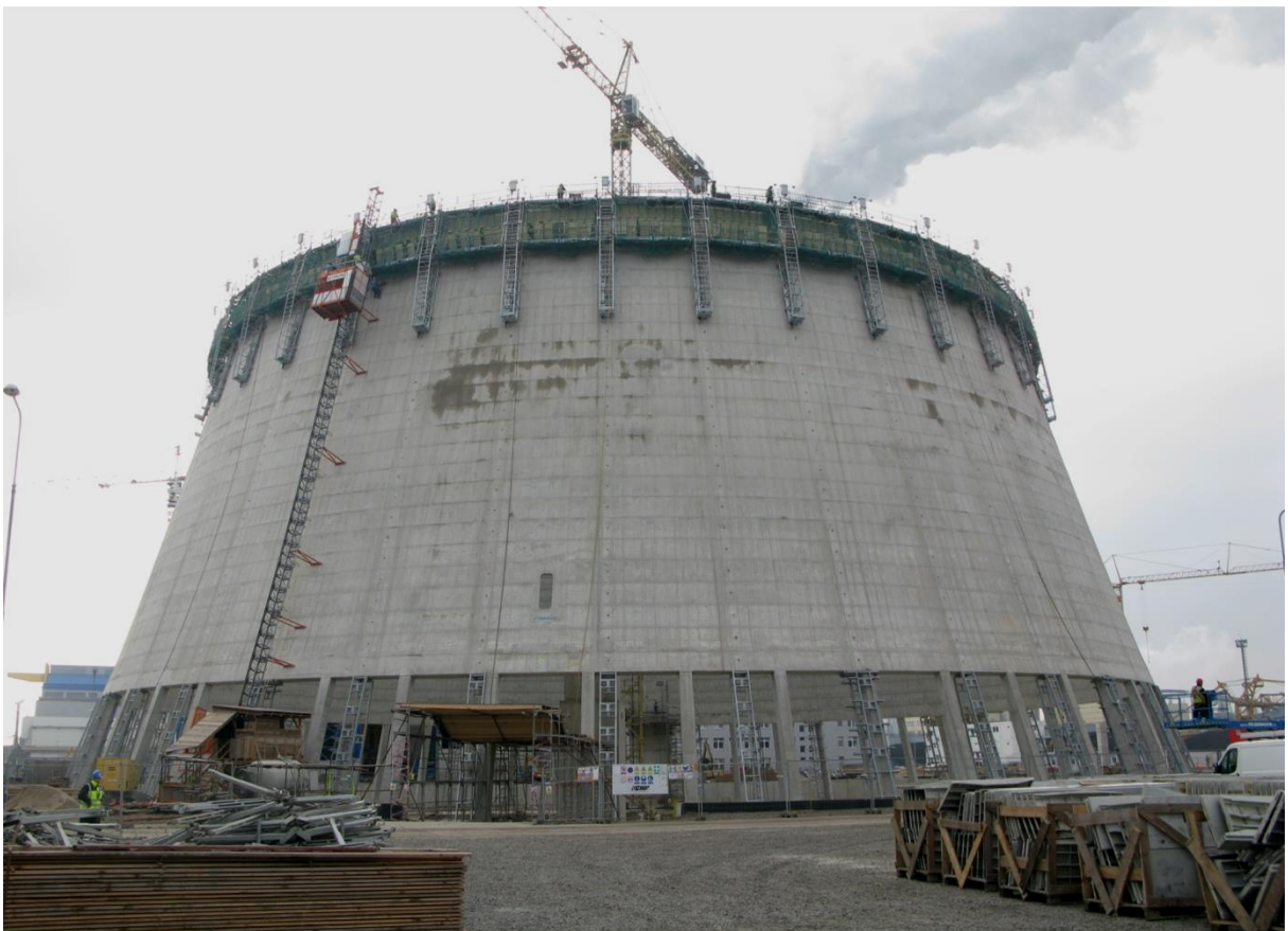
Figure 34 – Set of device – view of the passenger lift and temporary entrance into the tower
