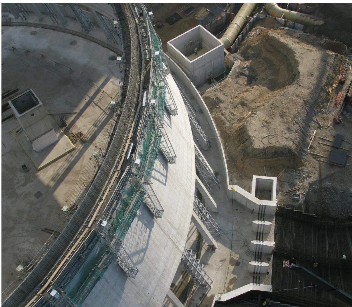
Figure 28 – Outlet channel and inlet pipes orientation
