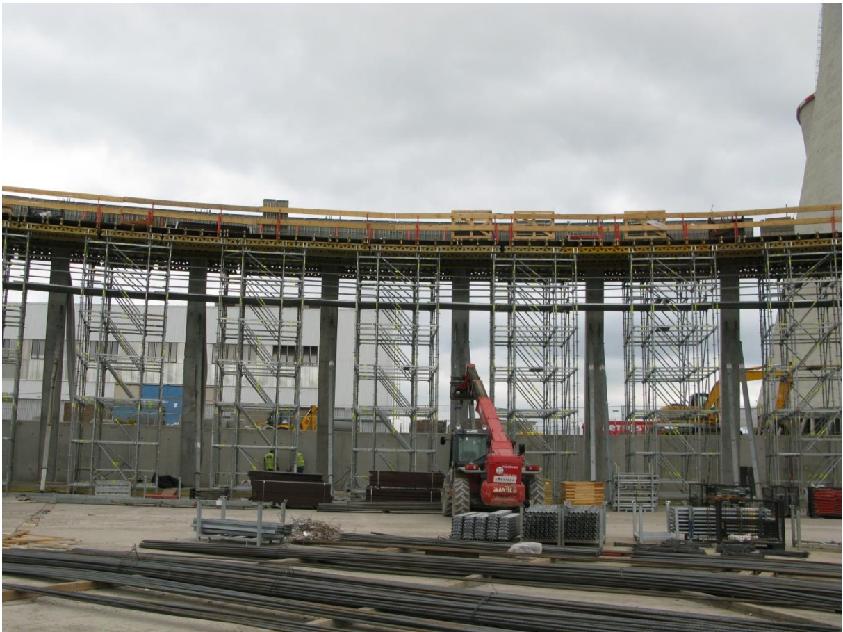
Figure 8 – First strap formwork
