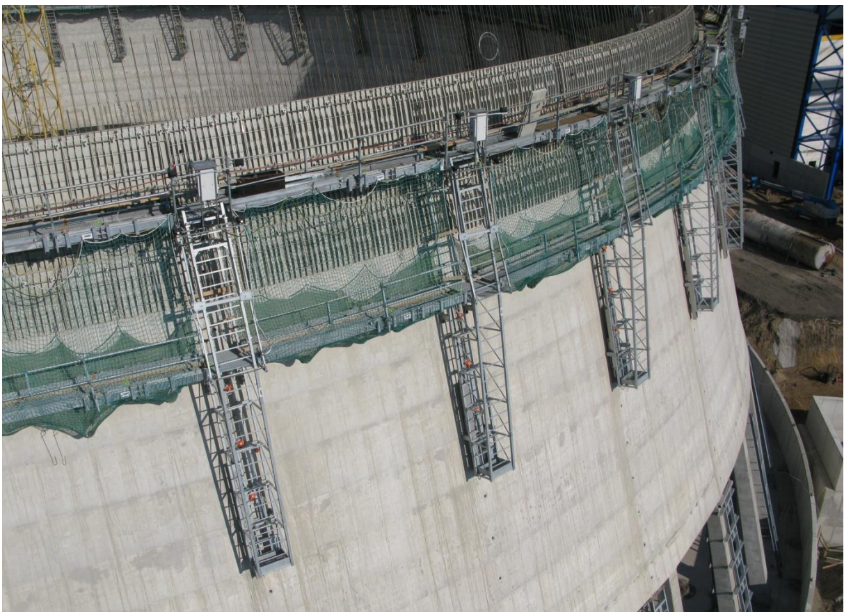
Figure 32 – Set of device together with formwork system and installed safety nets
