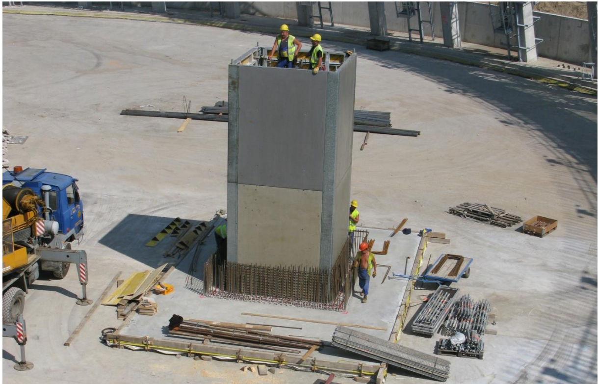
Figure 19 – Building the climbing channel
