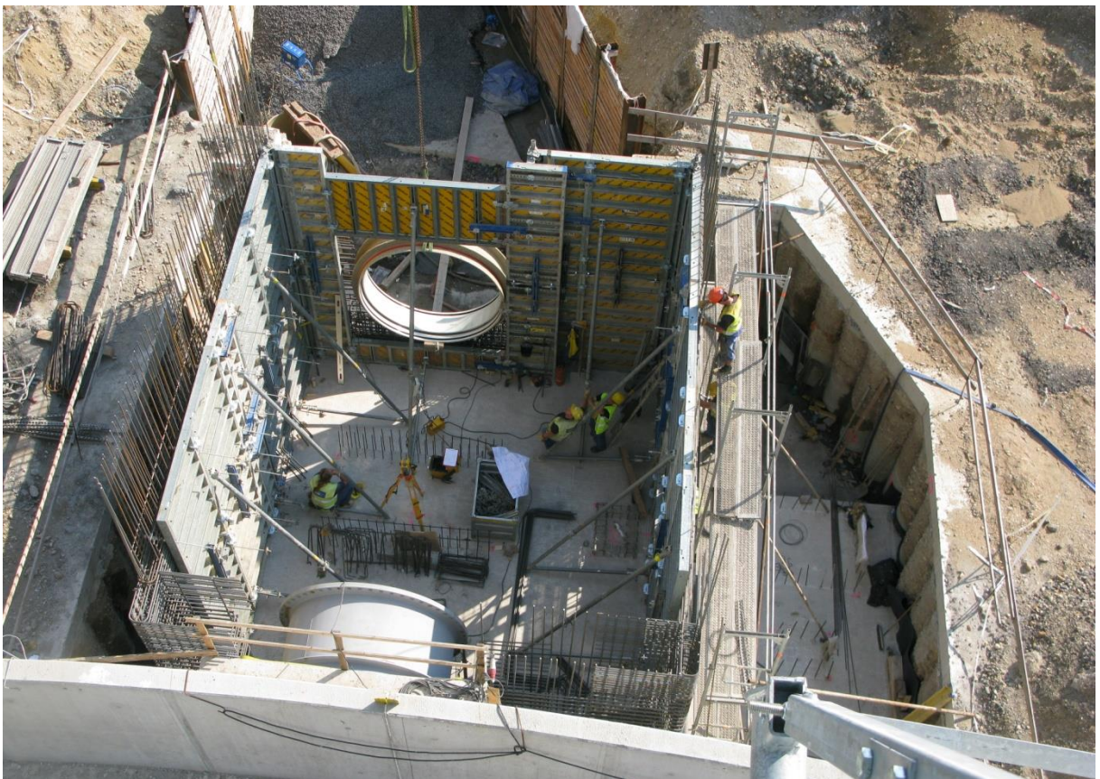
Figure 22 – Building the chamber to house the closing flap on the inlet channel
