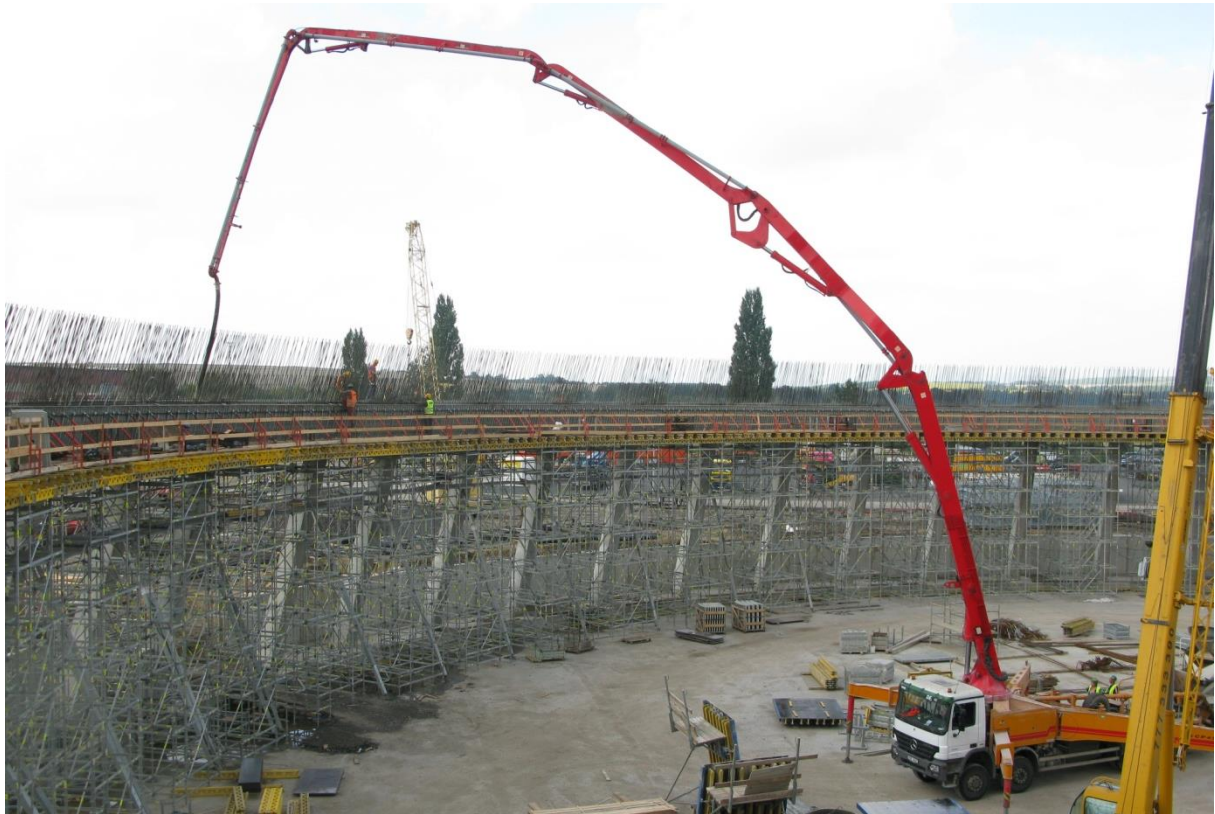
Figure 9 – Concreting the first strap (lead wing)
