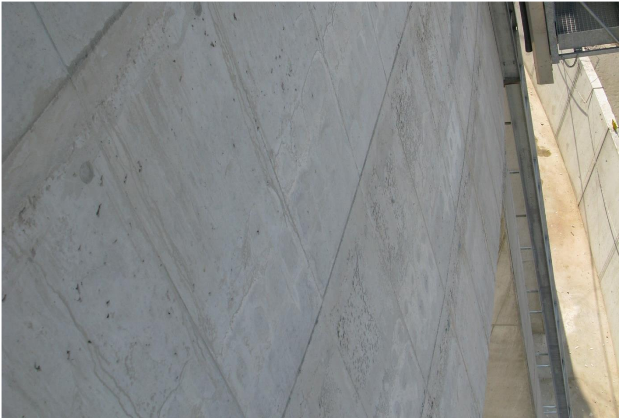
Figure 21 – The process results in very clean concrete aprons
