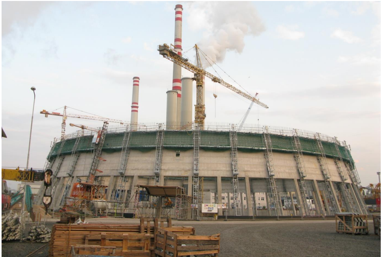
Figure 23 – Set of device prior to the concreting of the seventh strap
