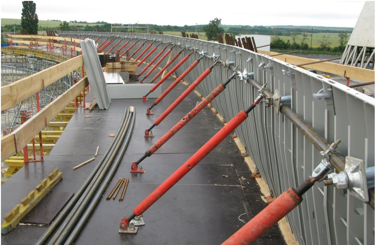
Figure 7 – First strap formwork (lead wing)
