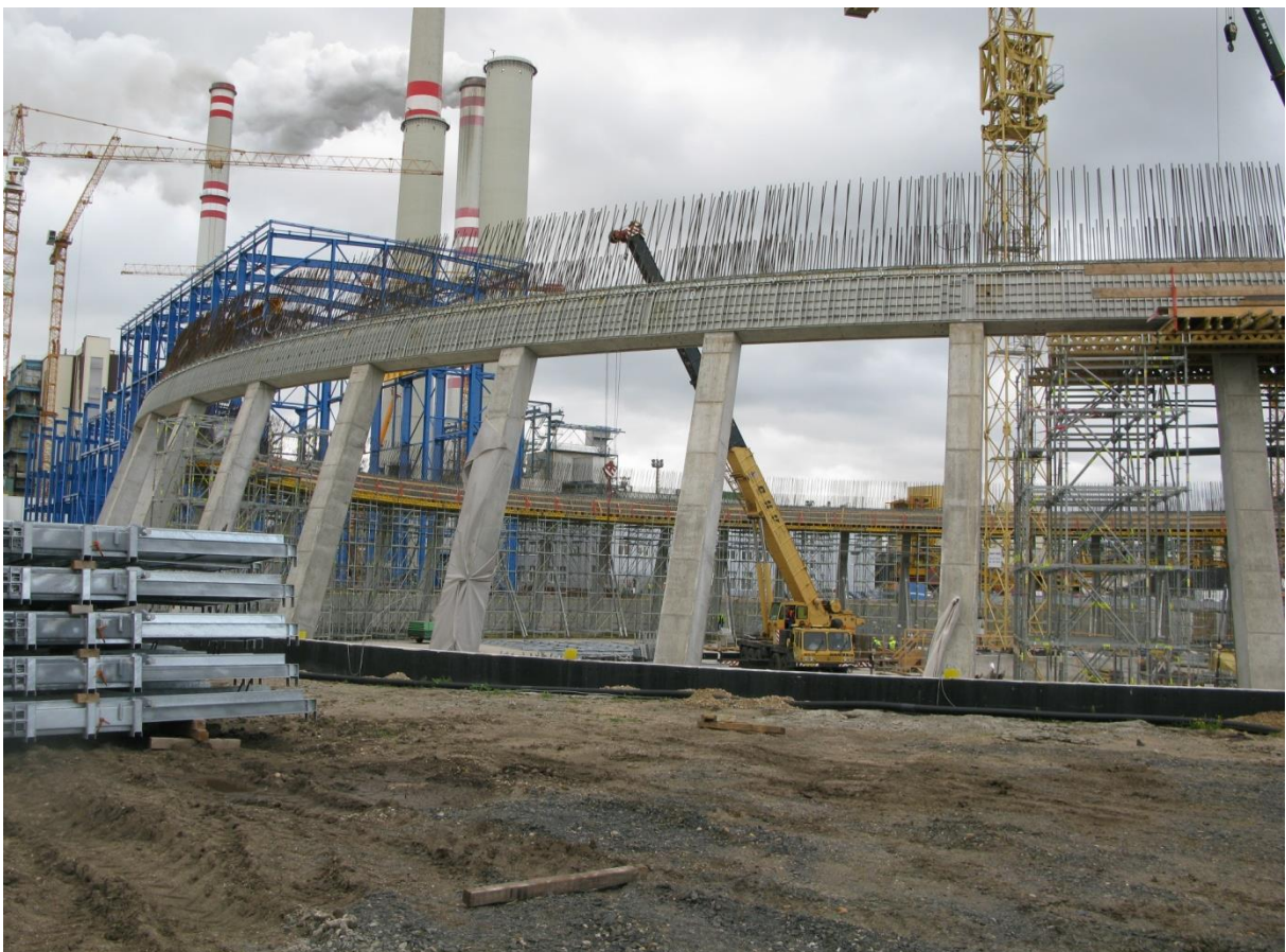
Figure 12 – First strap after the removal of support
