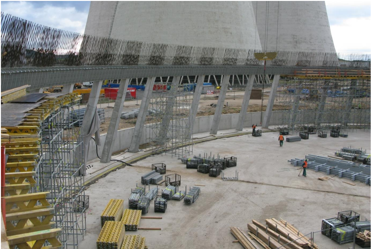
Figure 11 – Removing the first strap support
