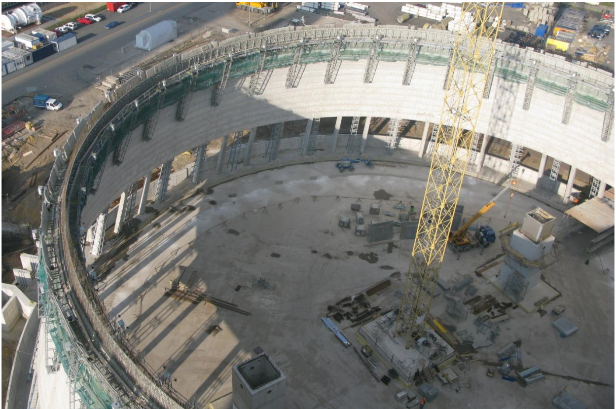
Figure 26 – Set of device during the concreting of the 15 th strap – formwork is getting in place
