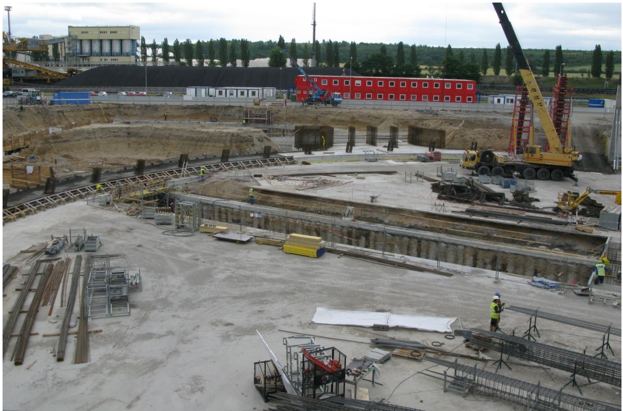
Figure 4 – Founding the tower columns
