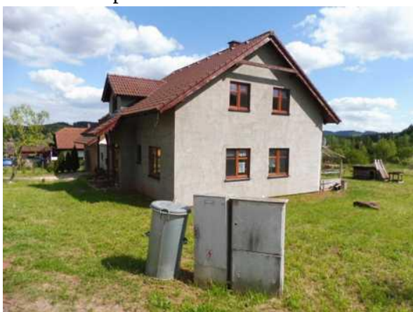
pilř el. energie
